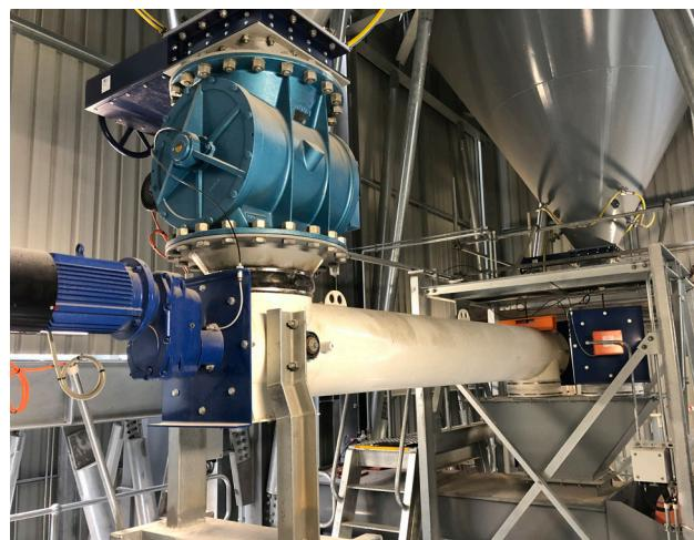
Accurate performance starts with thoughtful design. Screw diameter and speed are precisely engineered to ensure optimal material loading and maximise weighing accuracy. The achievable accuracy depends on both the product characteristics and the specific application.
